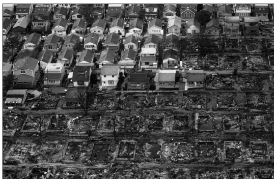
Top left: Pier in Seaside Heights, New Jersey, in the aftermath of Hurricane Sandy. Bottom: Burned houses are seen next to those that survived in Breezy Point.
